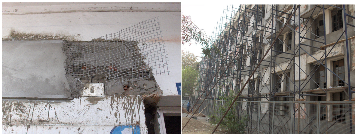
Figure 1. A seismic belt under construction (left); the exterior of the school (right)
