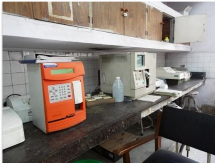
Figure 17: Table top medical equipment without anchoring or restraining
