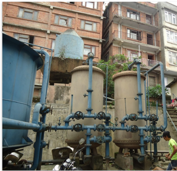
Figure 11: Rigid piping in sand filter tank (left); Rigid pipes in carbon filter, ammonia removal and softening tanks (right)
