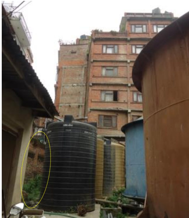
Figure 9: Unreinforced brick masonry boundary wall may topple due to out-of-plane forces and cause damage to the water storage tanks
