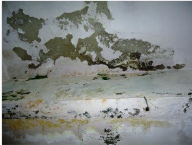
Figure 18: Seepage in the Emergency Laboratory
