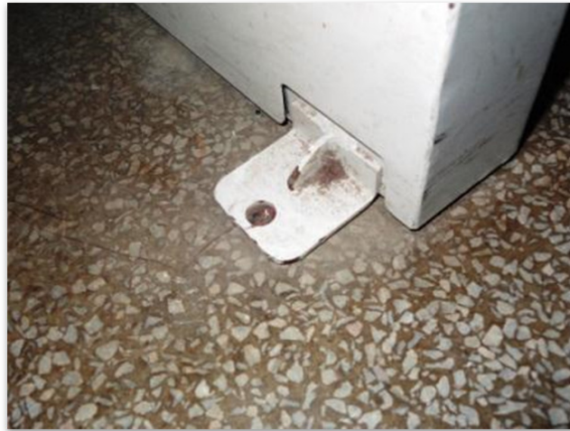
Figure 16: X-Ray machine bolted to the floor.
