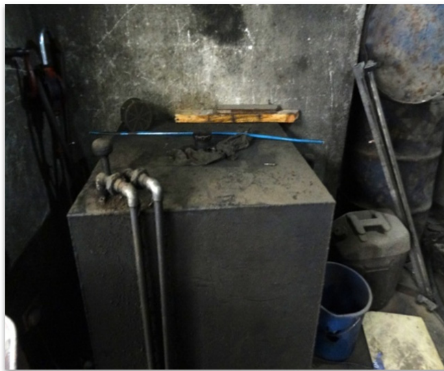
Figure 7: Generator fuel tank without flexible piping
