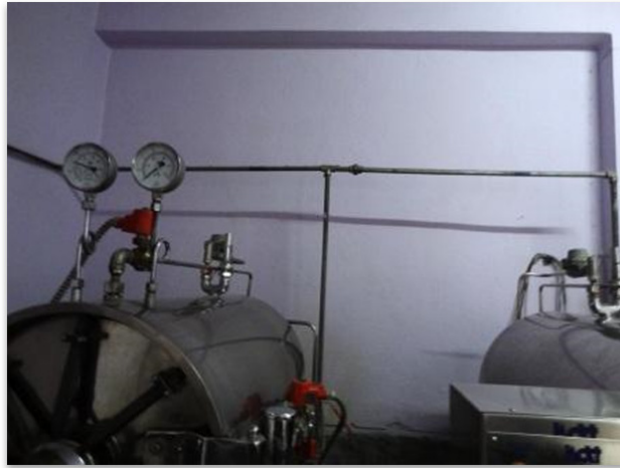
Figure 22: Rigid piping in autoclaves
