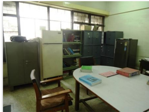
Figure 23: Unrestrained furniture and equipment susceptible to toppling and sliding
