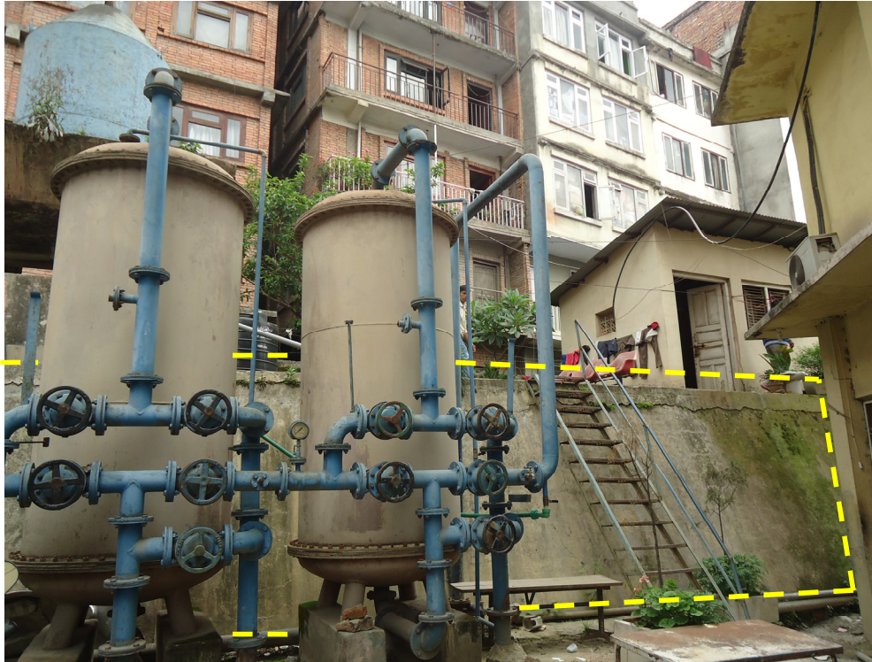
Figure 10: Ground level reinforced concrete water storage tank shown by yellow dashed line
