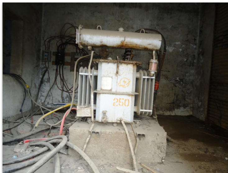
Figure 5: Transformer not secured to the concrete base
