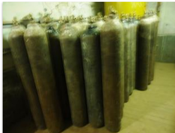
Figure 14: Unrestrained oxygen cylinder storage
