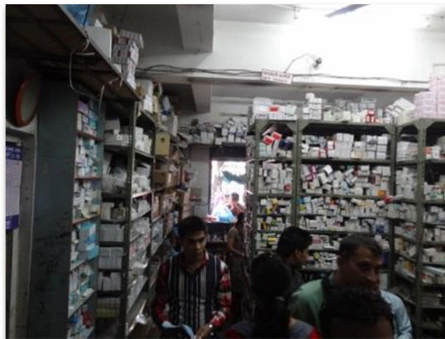
Figure 19: Unanchored shelves with unrestrained contents in the pharmacy
