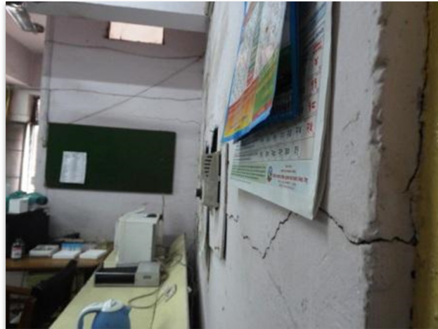
Figure 25: Infill walls with long continuous cracks in the Emergency Lab and Blood Bank
