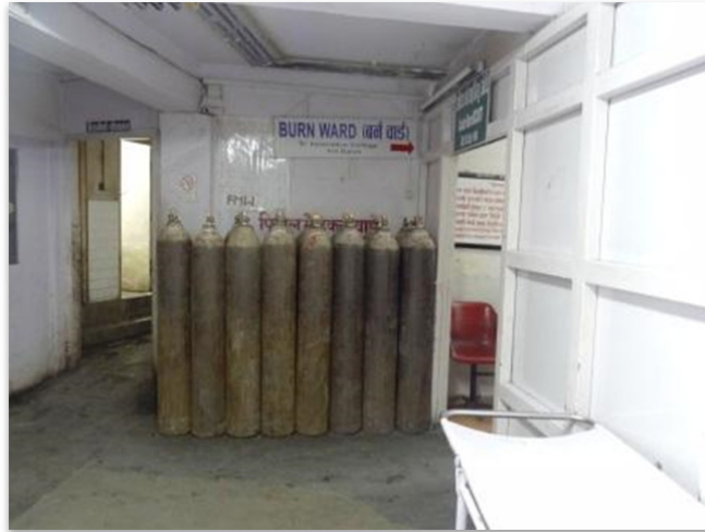
Figure 20: Unrestrained oxygen cylinders at the entrance to the Burn Ward
