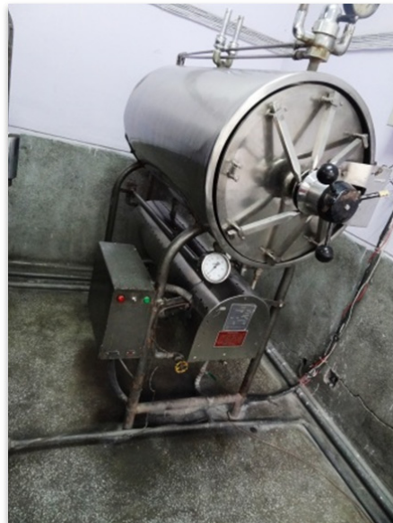
Figure 21: Autoclave in CSSD not bolted to floor or anchored to wall
