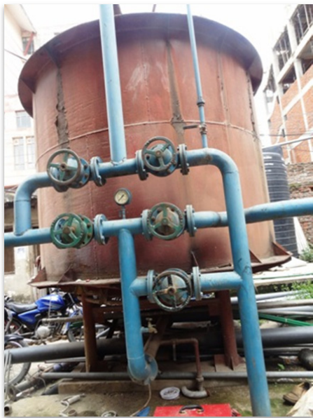
Figure 11: Rigid piping in sand filter tank (left); Rigid pipes in carbon filter, ammonia removal and softening tanks (right)
