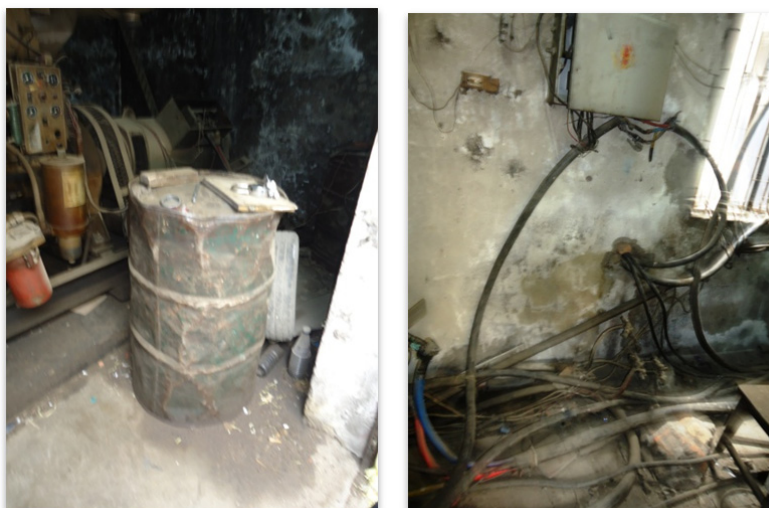
Figure 8: Reserve fuel drum without anchoring, susceptible to toppling and spillage and posing a fire hazard (left); No ducting or trays for electrical cables (right)
