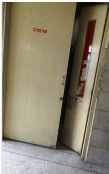
Figure 26: Narrower leaf of door kept open while wider leaf is kept shut
