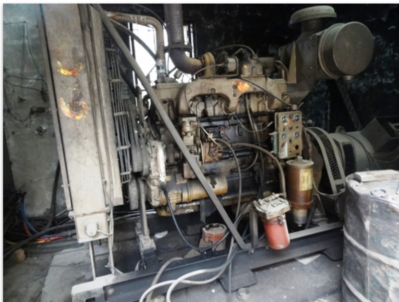
Figure 6: Generator without proper anchoring to the base plate
