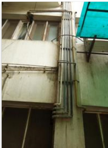
Figure 13: Lack of flexible connections at gas pipe bends
