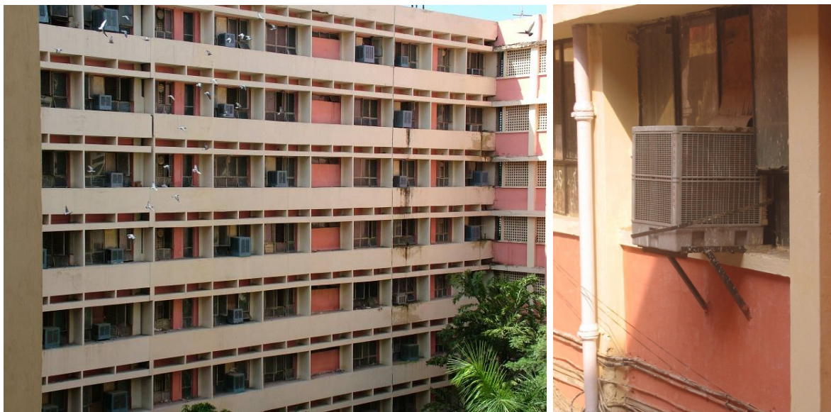
Figure 6. Elevation views of interior courtyard showing fins, cupboards (wide cream-colored bands) and air coolers (left); inadequately secured air cooler (right)
