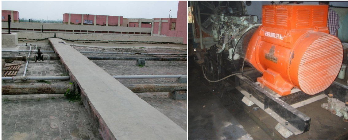
Figure 10. Rigid pipes crossing an expansion joint on the roof (left); unanchored emergency generator (right)
