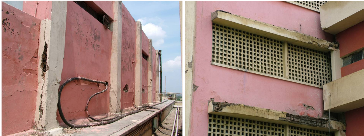
Figure 7. Corroded columns at machine room on roof (left); spalled concrete on exterior architectural elements (right)
