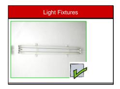
Tube lights can be secured to the ceiling with plastic clips. Screws should be used to secure the clips to the ceiling rather than self-adhesive pads.
