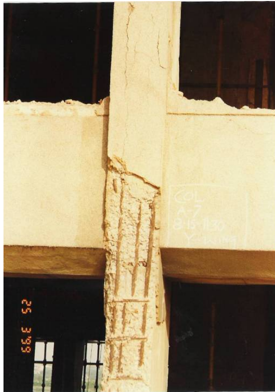
Figure 5. Column before rehabilitation showing tie spacing and deterioration
