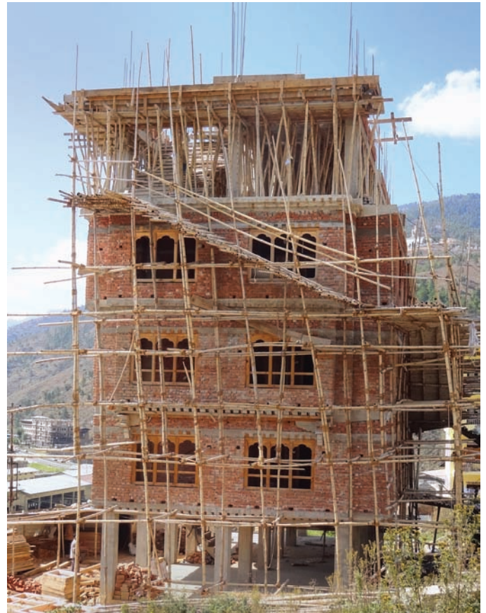
A building constructed with a concrete frame and brick masonry infill walls in Thimphu, Bhutan.
