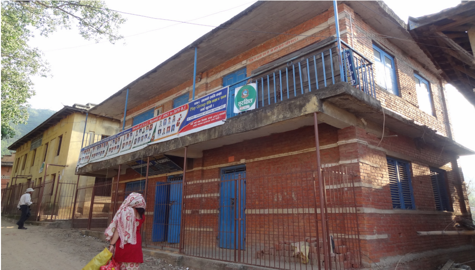
Green-tagged "Safe" in Nangkhel, Nepal: (L) the first school seismically retrofitted in 1997 through a program to train masons; (R) a new school built in 2000 by masons who had trained in the program. PHOTO: HARI KUMAR / EERI
