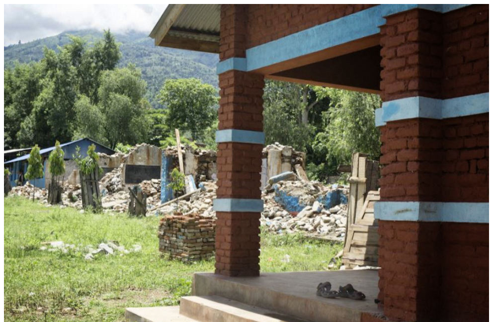
A library (right), built for earthquake resistance by Room to Read, stands next to the rubble of 6 unreinforced stone masonry classrooms that collapsed in Nuwakot, Nepal during the April 2015 earthquake. PHOTO: ROOM TO READ
